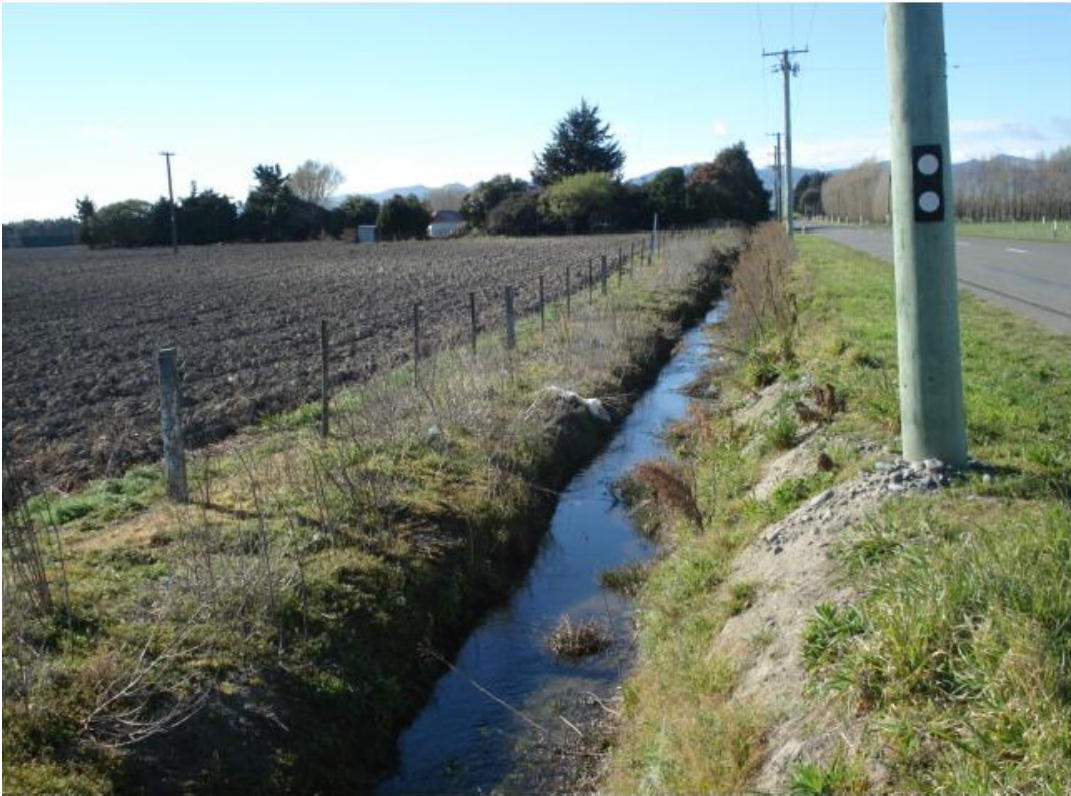
Figure 4; Existing Stockwater Race along Marshes Road
