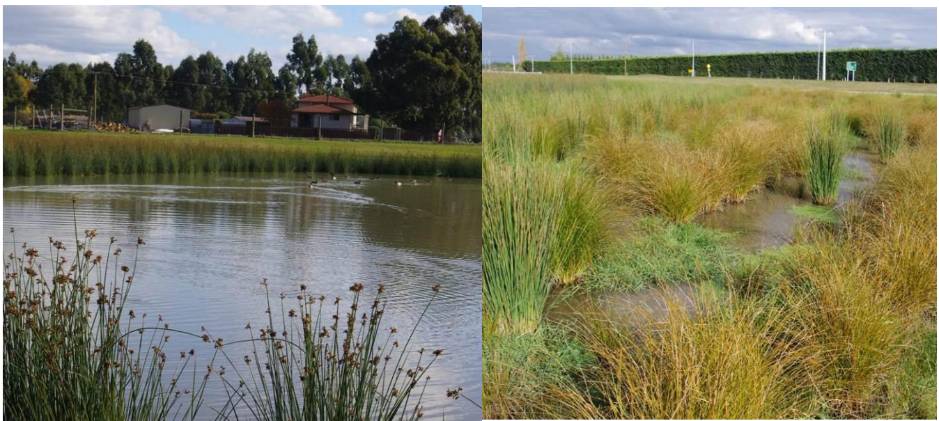
Photographs 17-18: Completed "Pond C" wetland
