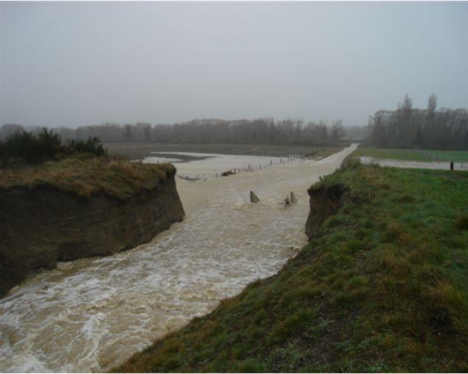
Photographs 1, 2: Wheatstone Drain in flood after the failure
