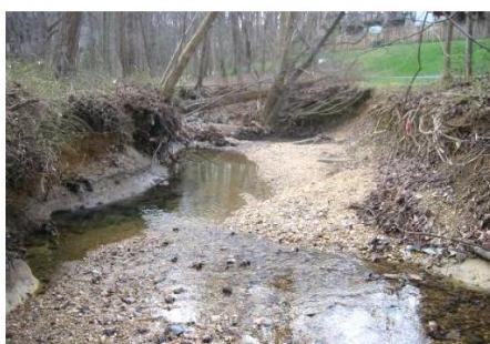
Photograph 2: Stream displaying effects of increased runoff and channel erosion.
