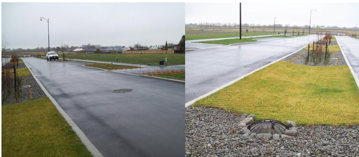
Figure 3: On-site stormwater management
