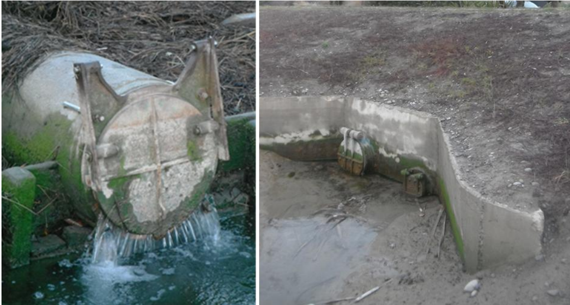
Photograph 3 and 4: Stormwater outlets draining to the Avon-Heathcote Estuary
