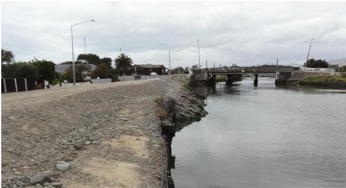
Photograph 1: Temporary stopbank on New Brighton Road, looking downstream toward Pages Road Bridge
