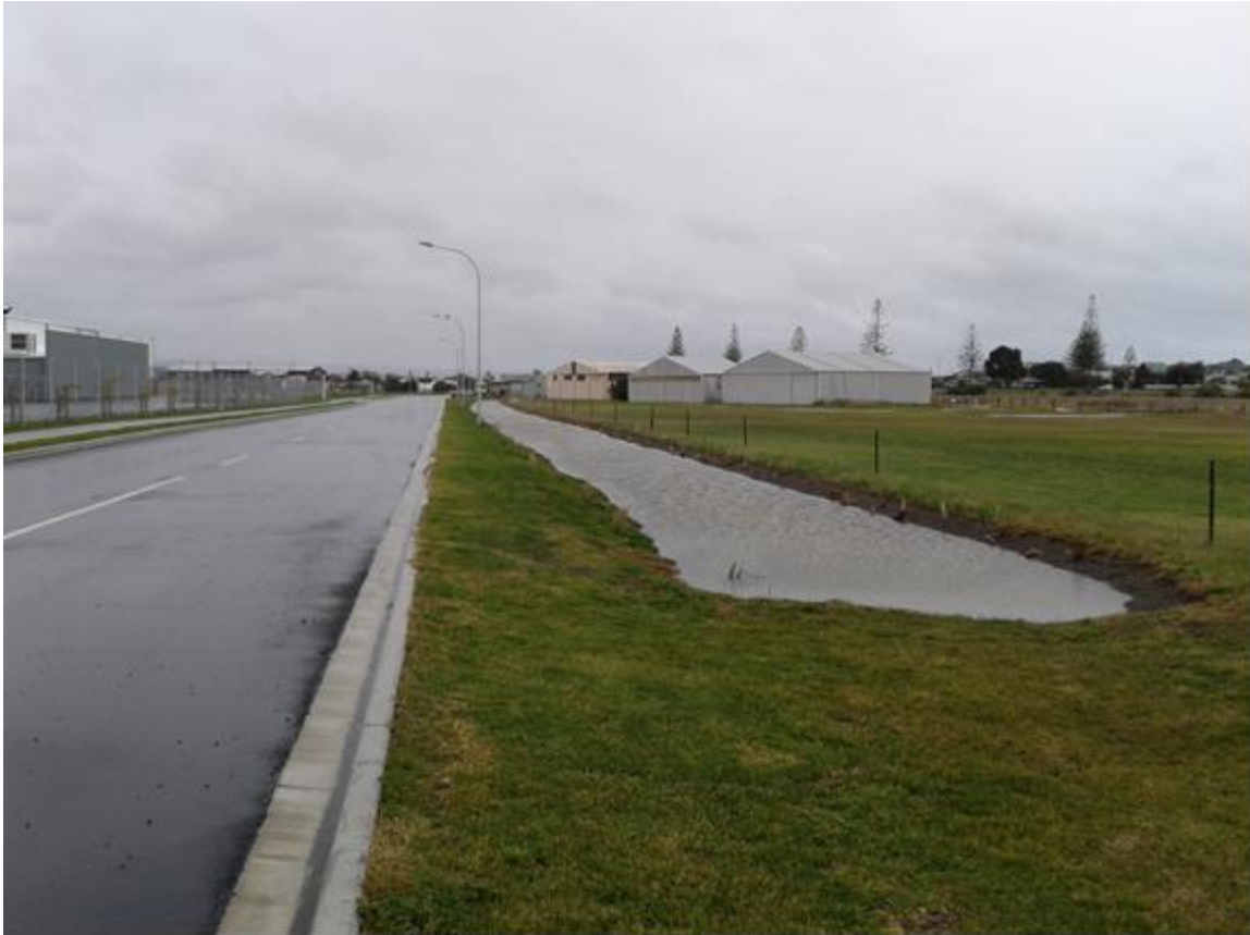
Photograph 5: Open Drain (Planting still to develop) in Wet Weather (July 2013)
