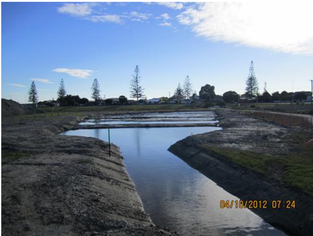
Photograph 3: Banded Wetland and Drainage Channel under Construction
