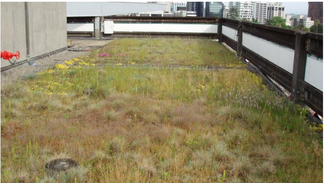
Photograph 2: Living roof designed specifically for stormwater mitigation, Faculty of Engineering building, University of Auckland, 2013
