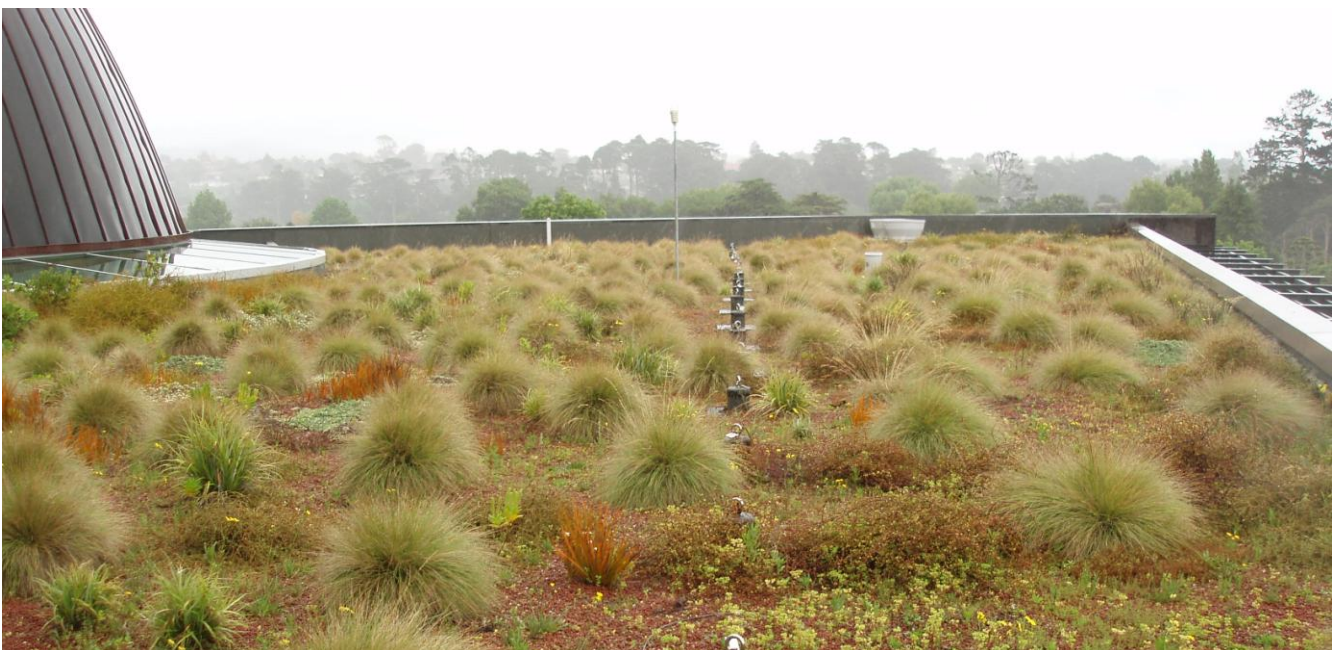
Photograph 1: Auckland Council Henderson Office Living Roof (December 2012)
