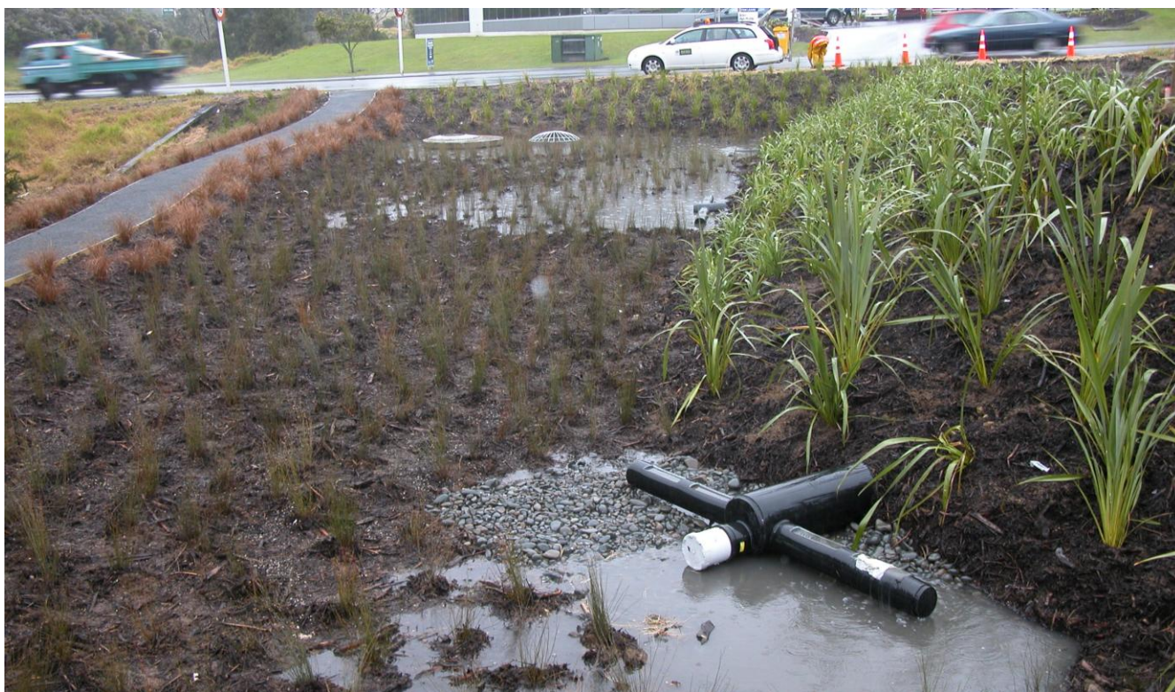
Photograph 2: Non-floating organic mulch placed over the bulk of a rain garden and stone mulch used in areas around stormwater inflow points, North Shore
