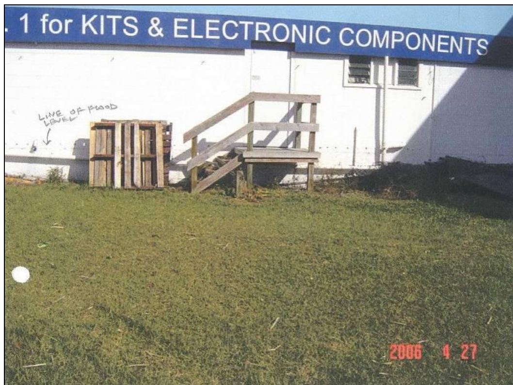
Figure 6: Photo showing the flood level from the April 2006 storm (dotted line). Note the flood level is marginally higher than the entrance level of this Wairau Rd commercial building.
