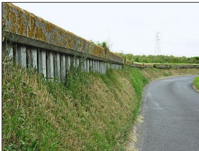
Photograph 3: Days of continually increasing flood protection heights could be numbered on.
