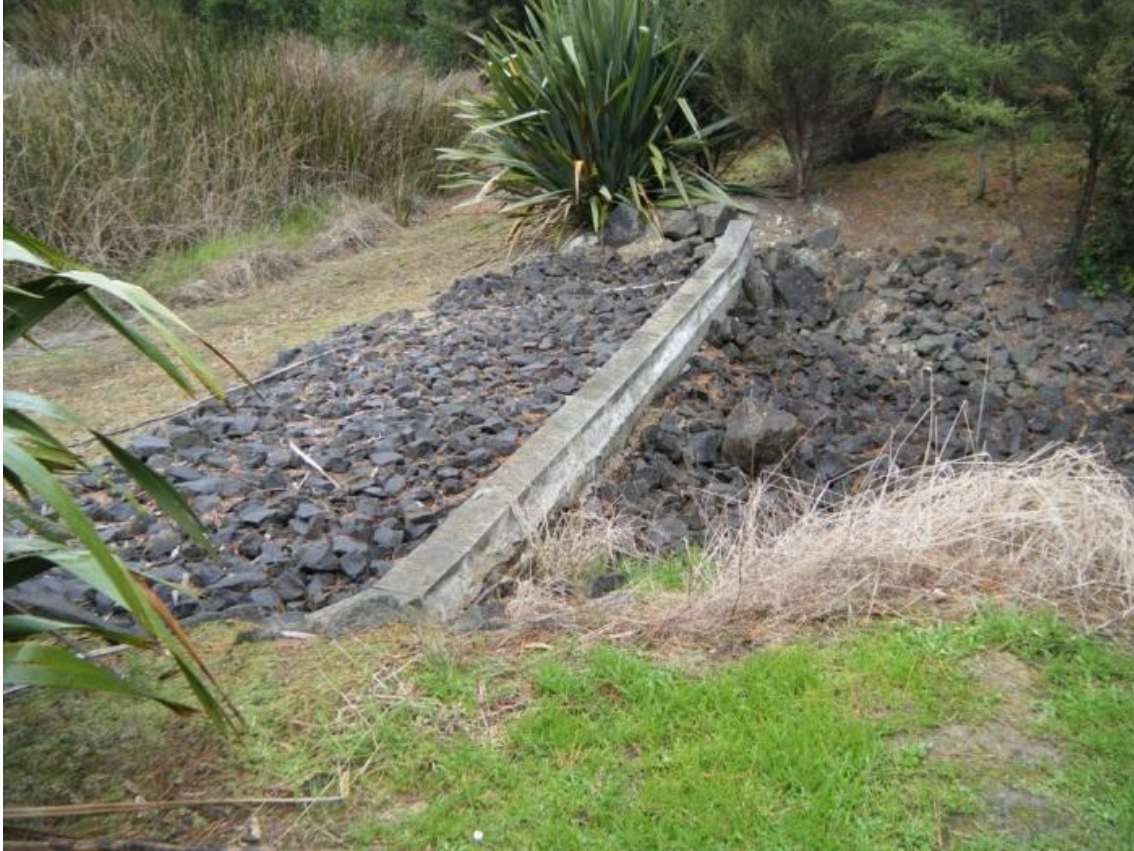
Figure 4 Well Designed and Constructed Concrete Beam Level Spreader
