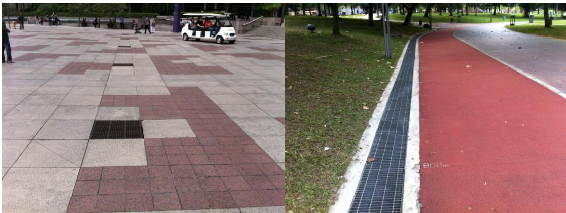
Figure 1 Redundant designs of catchpits in an overseas city
