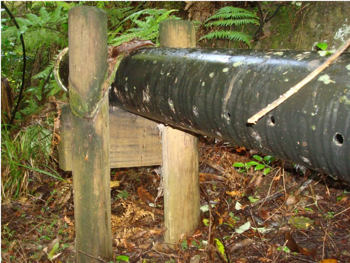
Figure 3 PVC pipe dispersal bar with timber supporting structure and outlet holes
