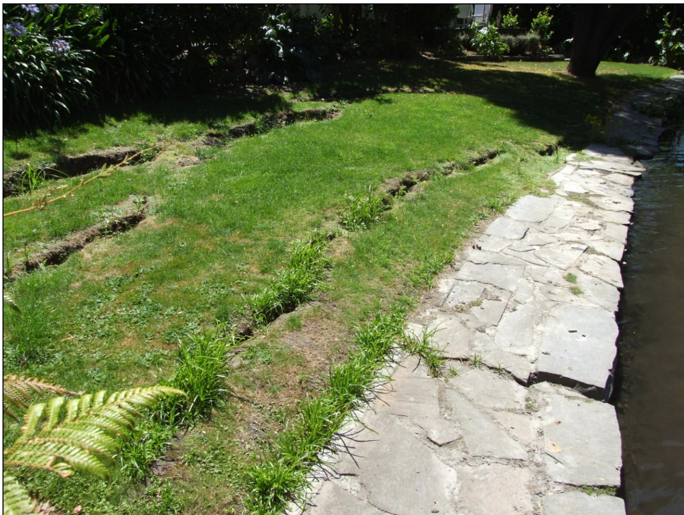
Figure 3: Earthquake related stream bank damage – Lateral Spread
