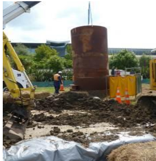
Fig. 18 Installing the steel casing
