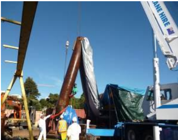
Fig. 24 Liner Insertion
