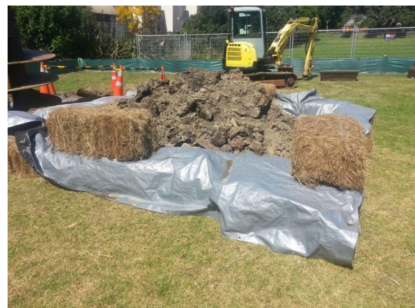
Fig. 20 Contaminated soil management
