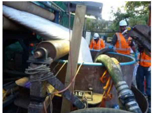
Fig. 27 Impregnated liner fed into the culvert
