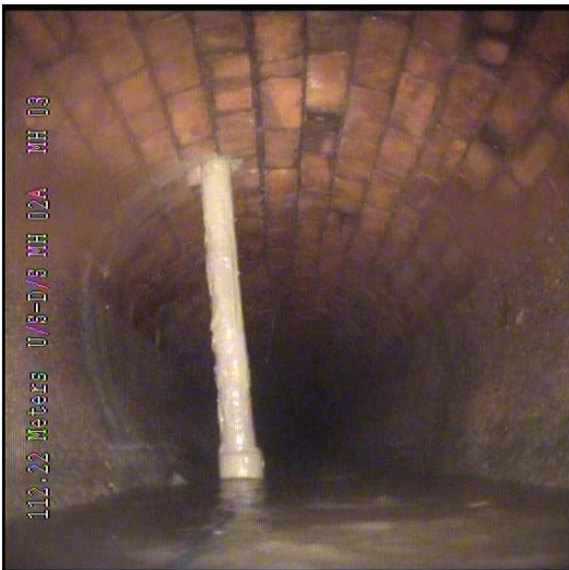
Fig. 17 Establishing the centre of the culvert
