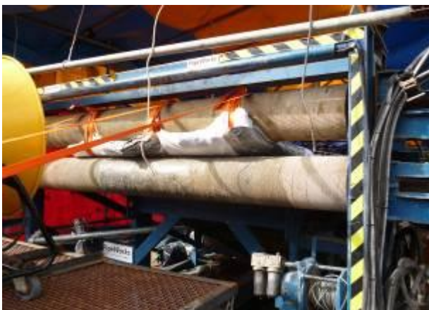
Fig. 22 Sealed Liner laid out on the roller system
