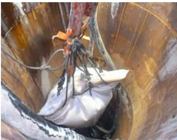
Fig. 26 Liner inversion setup, top of access shaft
