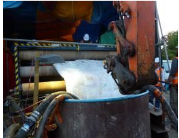
Fig. 25 Liner running to inversion chute
