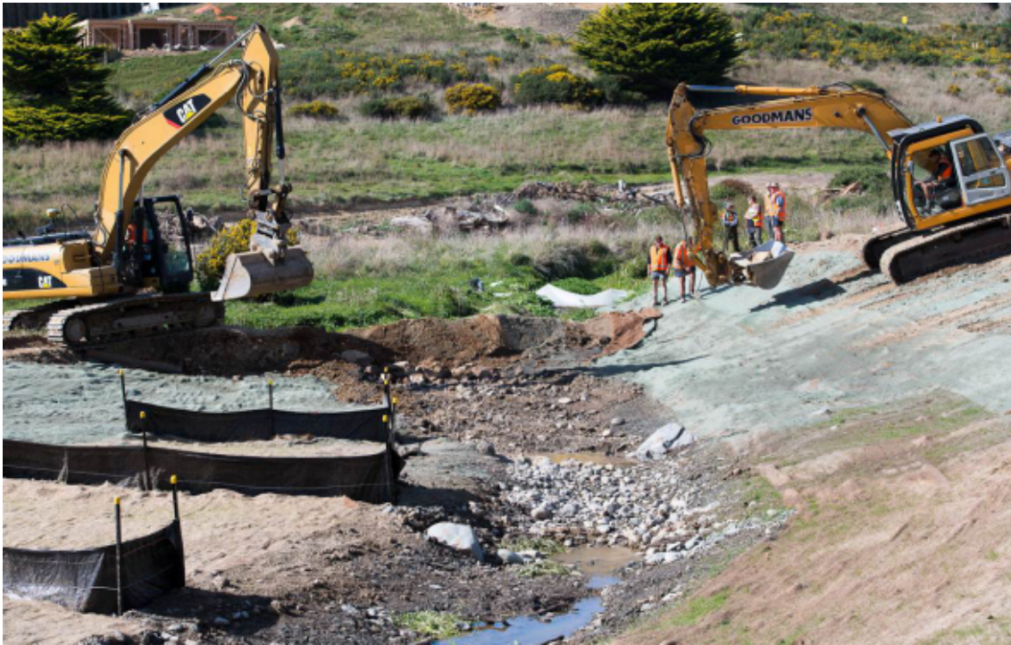
Figure 17: Duck Creek Diversion 1 Commissioning
