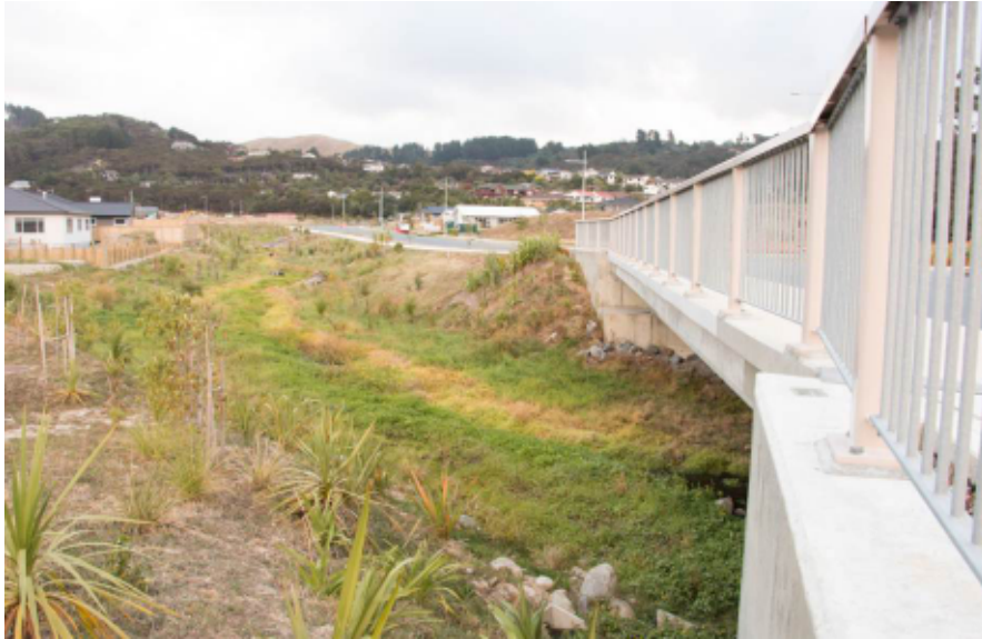
Figure 12: The Banks Resolution Drive bridge
