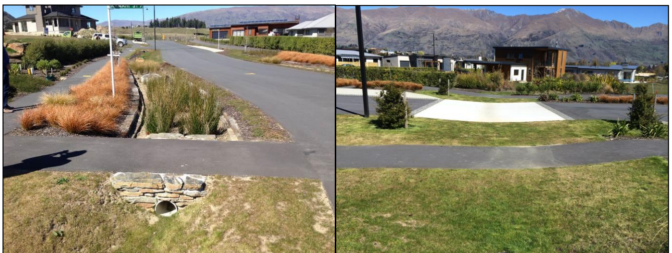
Figure 6. Kirimoko Park WSUD Design Elements (on left is a raingarden and swale and on the right, a swale-to-ford footpath and road crossing)
