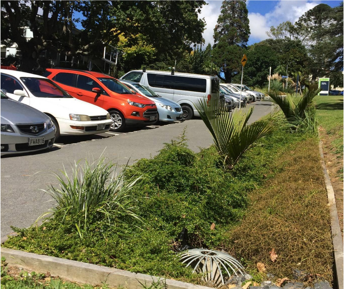
Photo 2: Road-side swale – entry under footpath
