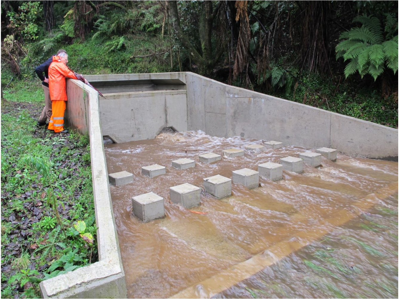
Figure 4: Outlet Structure during 5 year event
