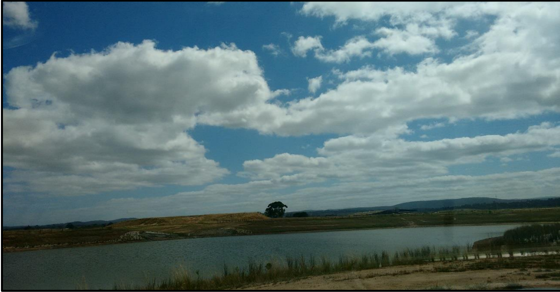
Figure 2-4: Southern Storage Dam (24th February, 2015)
