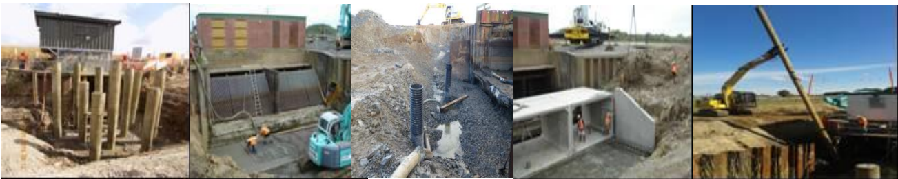
Photograph 11 Foundation works during construction
