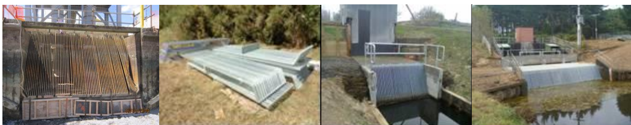
Photograph 2 Inlet bays showing old and newly installed screens
