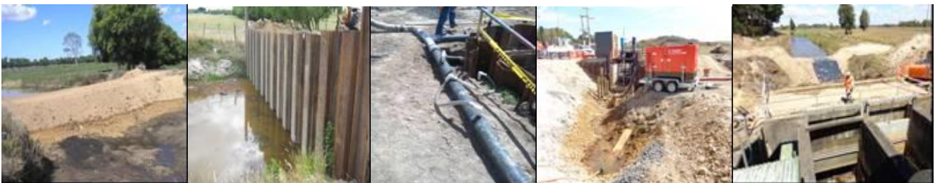
Photograph 10 Cofferdams and dewatering during pumpstation upgrade
