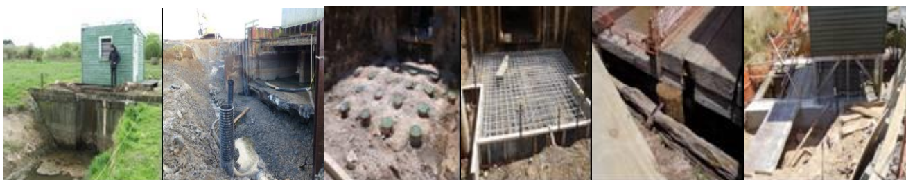
Photograph 3 Old and rebuilt sumps
