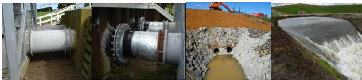
Photograph 8 Installed gibaults and outlet protection works
