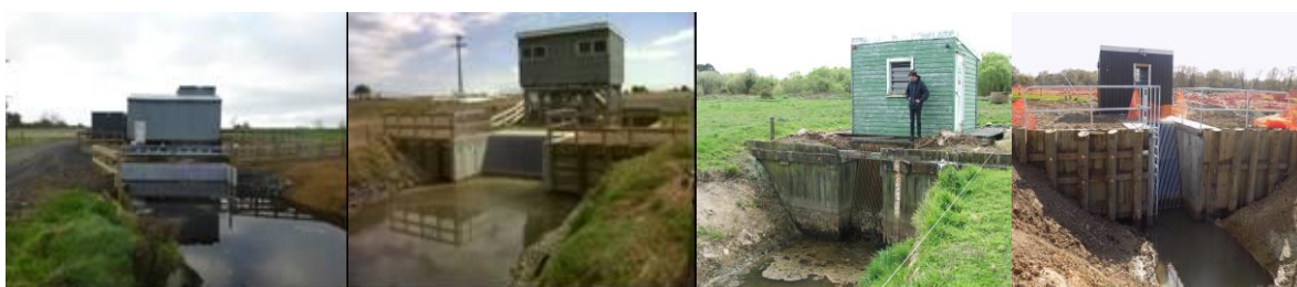
Photograph 9 Existing and new pump sheds
