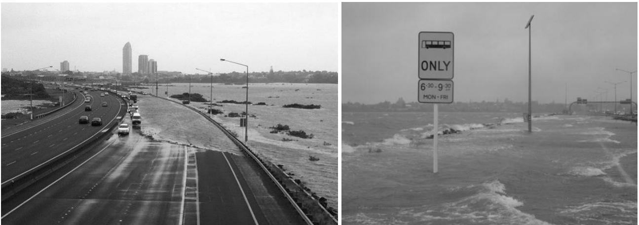
Figure 1: Flooding in Shoal Bay near Northcote (left) and on the Auckland north-west motorway (Metservice archive).
