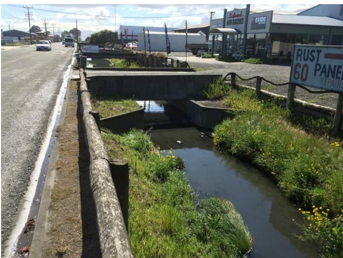
Photograph 7: Beach Road Drain with Bridge Constrictions Fills to Capacity
