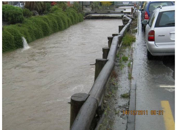
Photograph 7: Beach Road Drain with Bridge Constrictions Fills to Capacity
