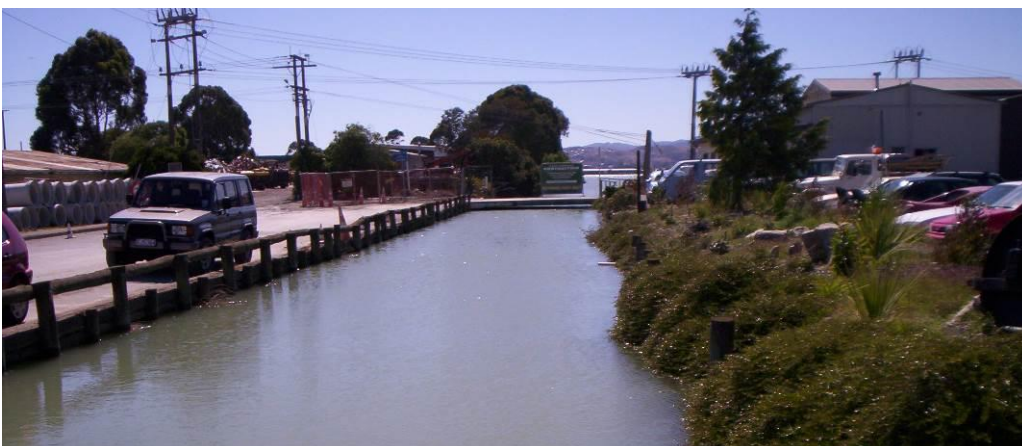
Photograph 8: Beach Road Drain Outlet During a King Tide
