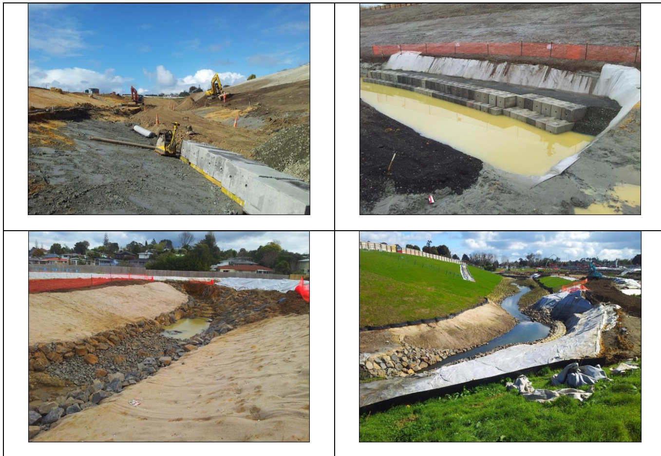
Figure 9: Photographs of the realigned section of Oakley Creek under Construction
