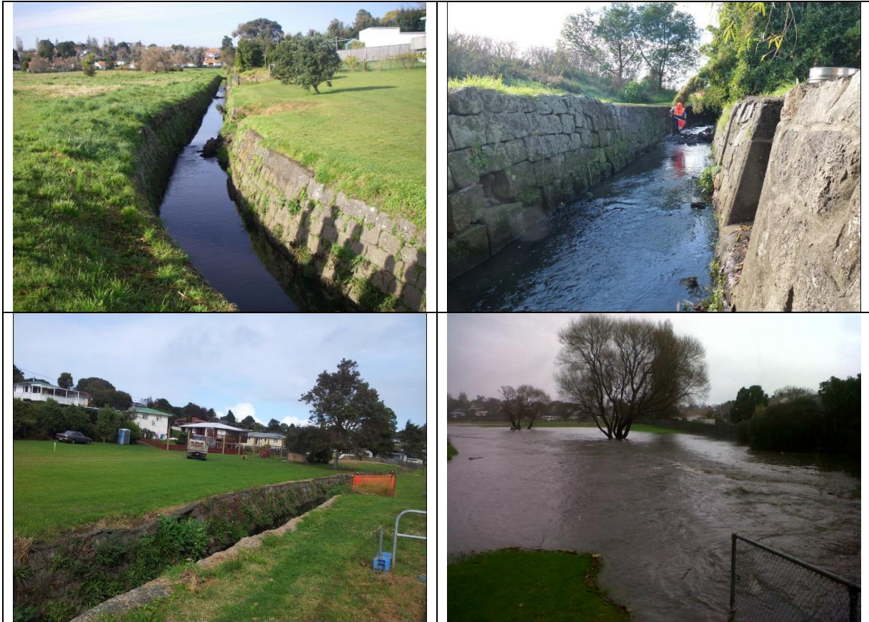
Figure 7: Oakley Creek in Alan Wood Reserve showing basalt rock wall channel sections, Flooding downstream of Richardson Road culvert on 1 June 2010 after rainfall equivalent to 1 to 2 year ARI rainfall intensity
