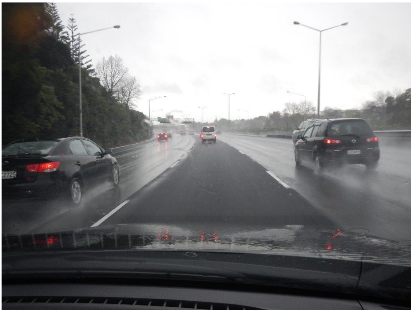
The spray suppression benefit of fresh open graded porous asphalt (OGPA)
