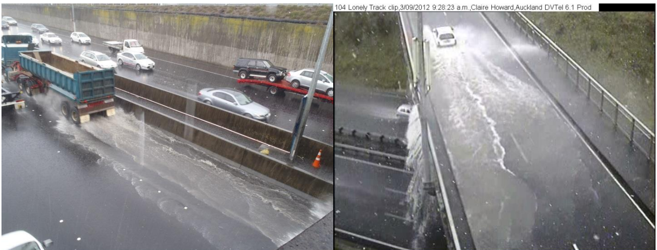
Stormwater surface flooding presents safety risks to motorists
