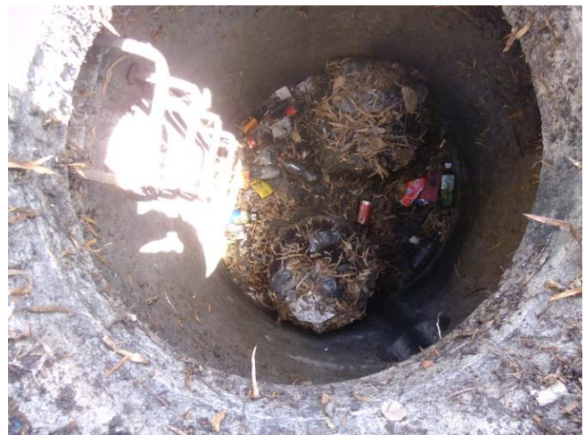
Figure 6: Gross Pollutants in Soakhole
