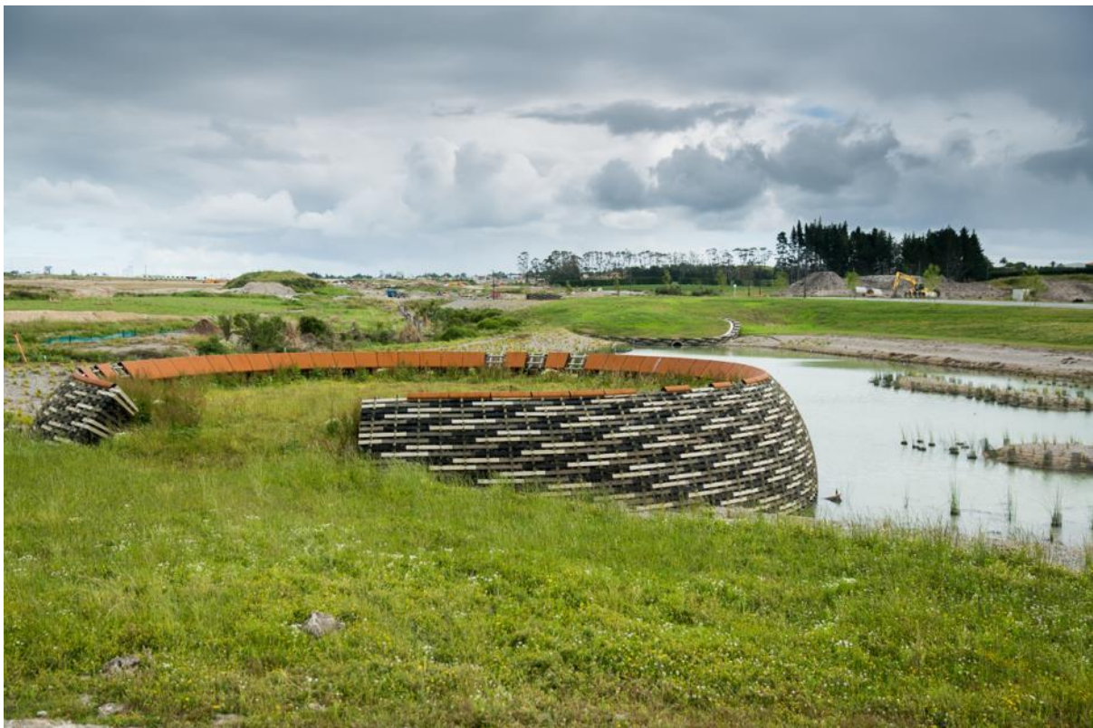
Figure 10. Kopupaka Park under construction.
