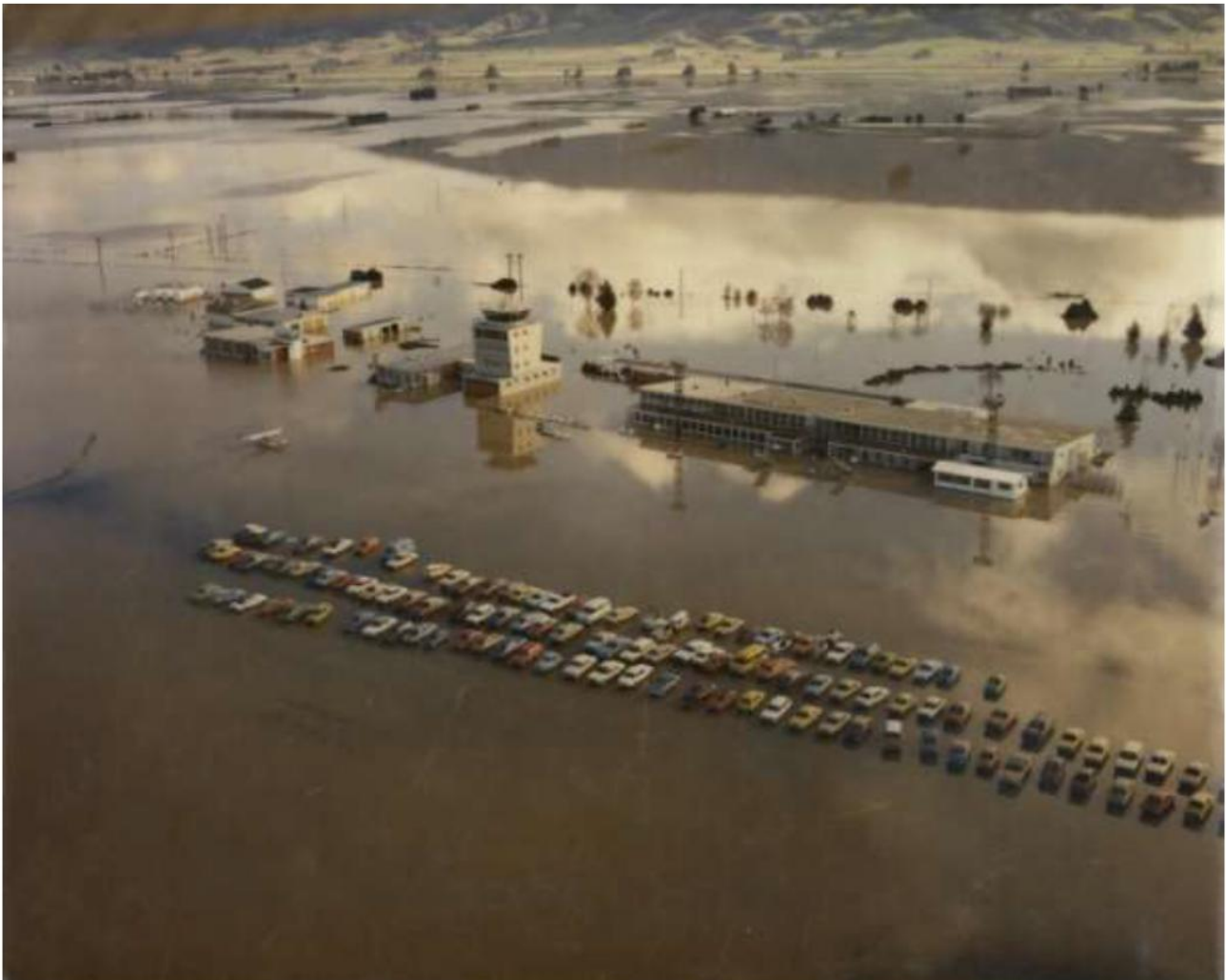
Photograph 1: Dunedin International Airport, during the June 1980 flood (Adapted from Natural Hazards on the Taieri Plains, Otago (p.12) by Otago Regional Council, 2013.)
