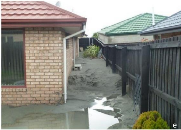
Figure 1 Observed liquefaction-induced land damage and dwelling foundation damage due to Christchurch earthquakes (from van Ballegooy et al 2014)
