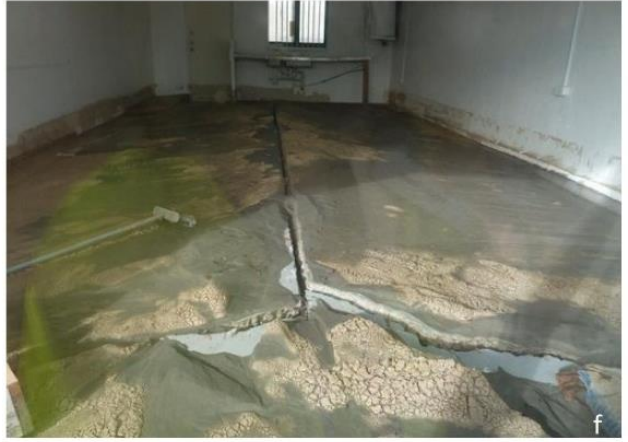
Figure 1 Observed liquefaction-induced land damage and dwelling foundation damage due to Christchurch earthquakes (from van Ballegooy et al 2014)
