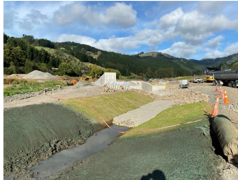
Stream diversion day
