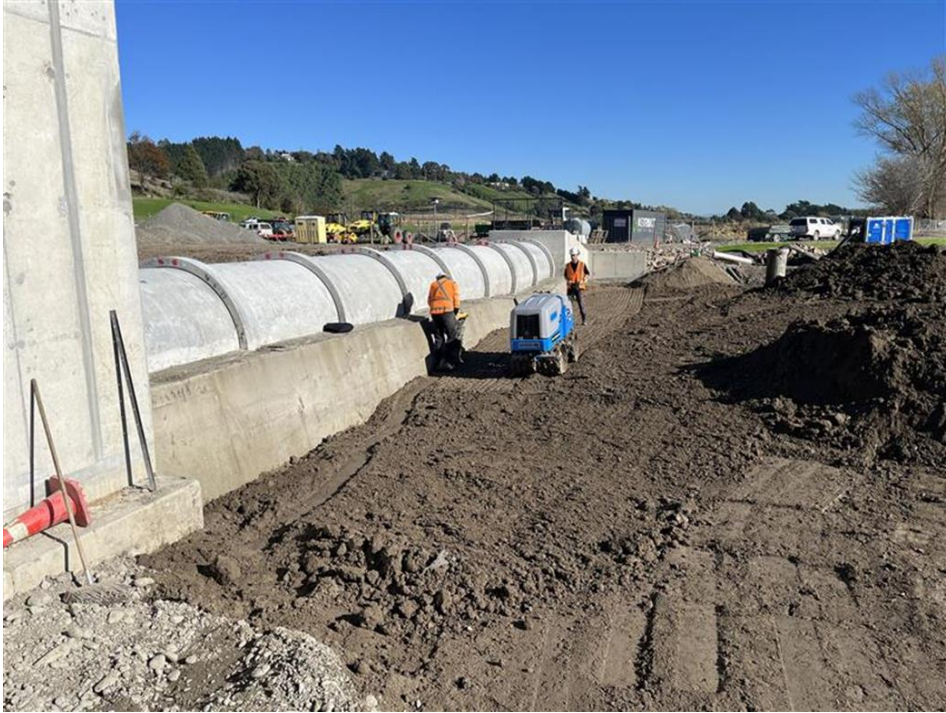
Compaction of Cashmere interface fills
