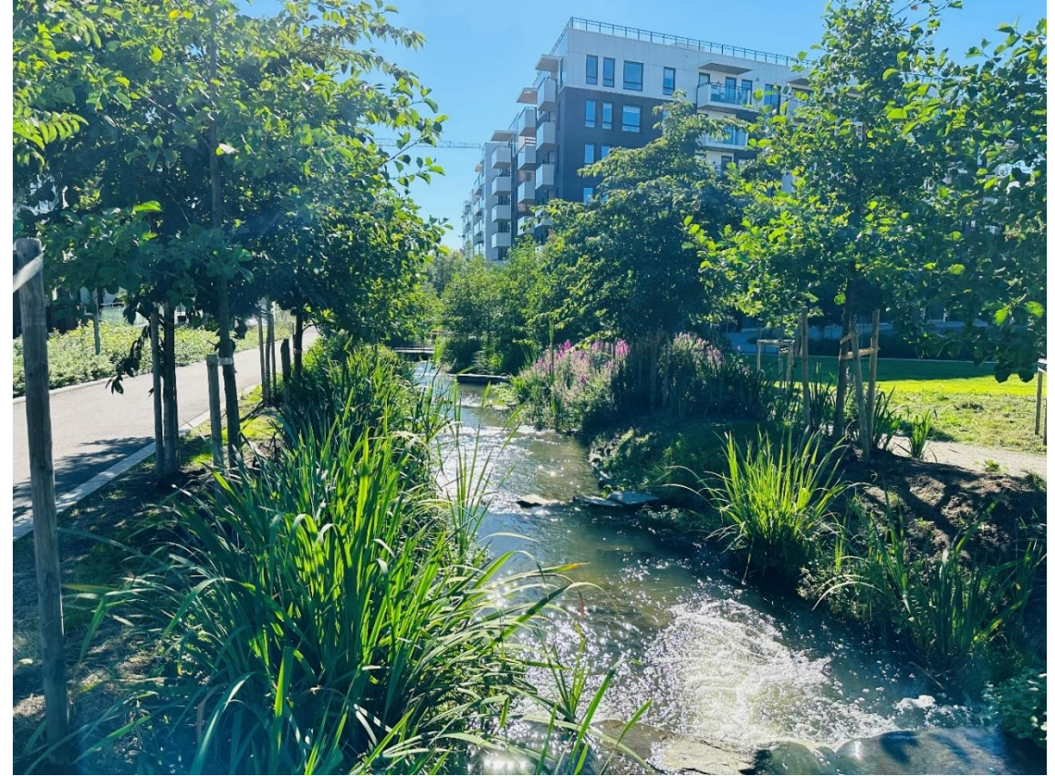
Oslo – daylighted stream conveying stormwater diverted from the combined system
