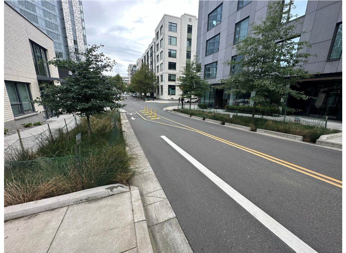
Fenced rain gardens
