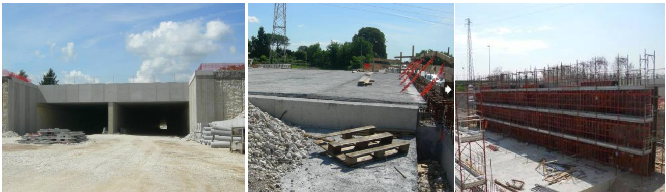
Figure 17: Pedemontana Veneta building yards
