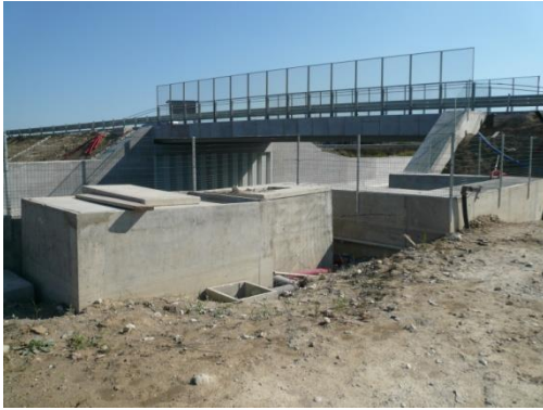
Figure 14: under construction filtration plant
