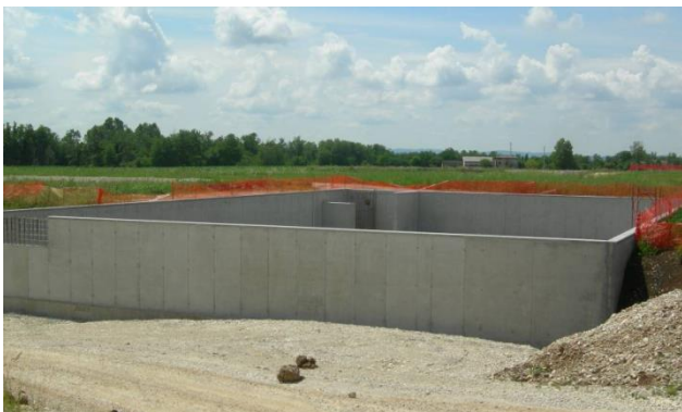
Figure 20: under construction detention basin
