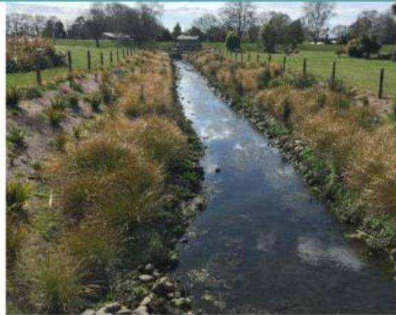
Banks planted with vegetation for stability, sloped sides to avoid slumping
