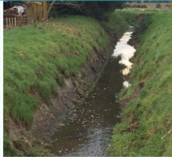
Vertically cut banks slumping into the base of the waterway
