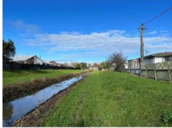
Clear of sediment build-up, sloped sides, mowed grass
