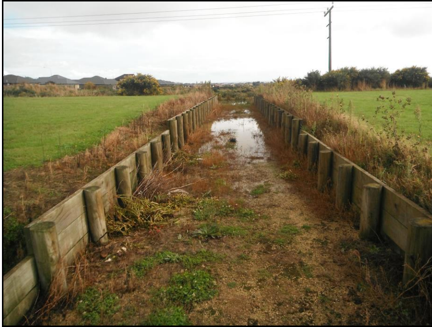
Figure 3: Walkway Secondary Overland Flowpath – Taken from Monaco Grove and Looking Towards the Johnstone Drive Gully
