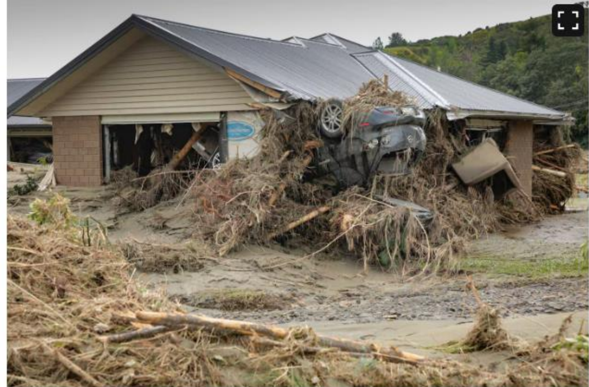
Michael Fowler says that based on the photos and information he had seen from Esk Valley after Cyclone Gabrielle, this flooding was worse than in 1938. Photo / Warren Buckland.
