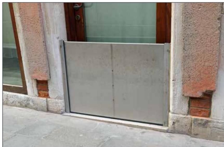
Permanent doorway flood panel
