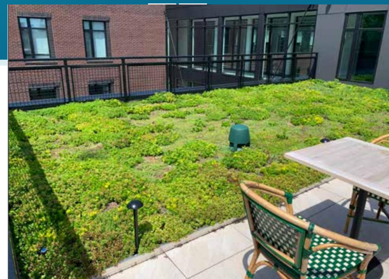
Vegetated green roof
