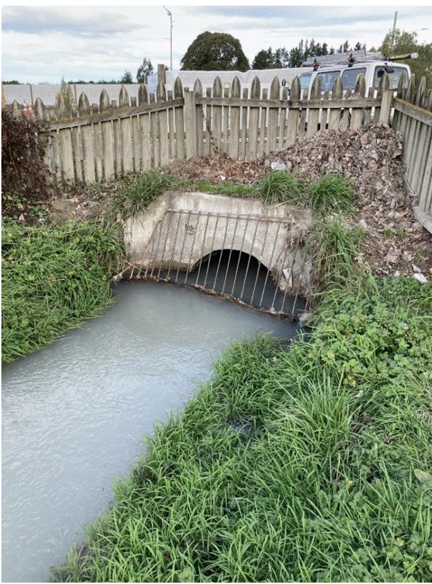
Plate 9: Existing 900 mm steel Armco pipe inlet
