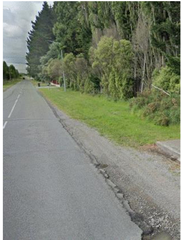
Plate 16: Weedons Ross Road grassed roadside channel
