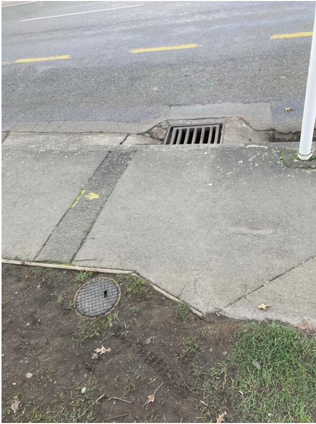
Plate 11: Existing sump to soak pit system
