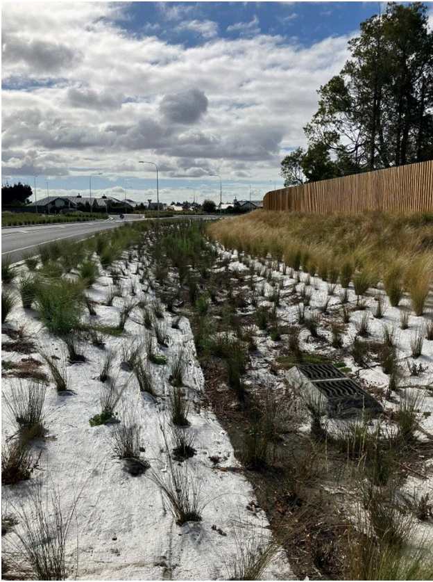
Plate 25: First-flush swales adjacent new link road
