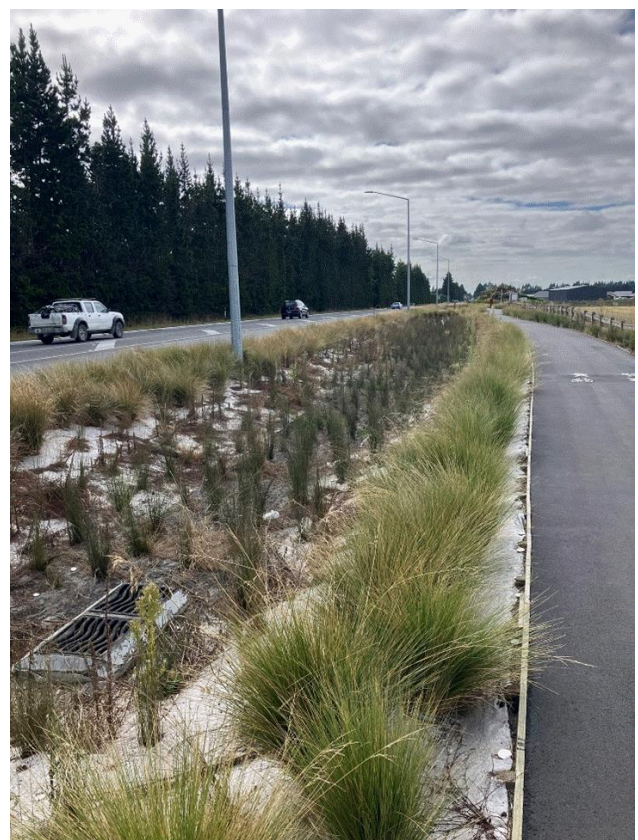
Plate 24: First-flush swales adjacent SH73
