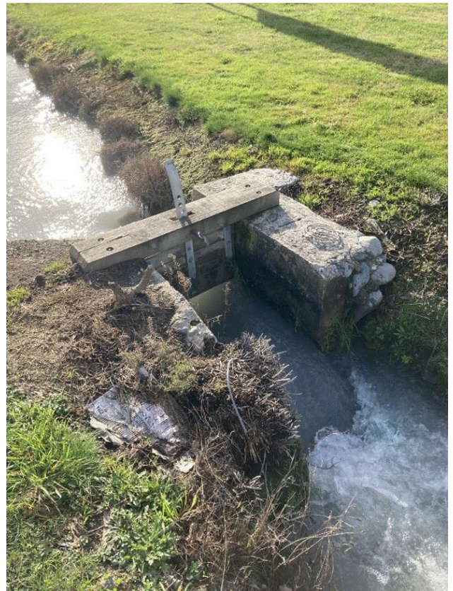
Plate 6: Existing stoplog gate
