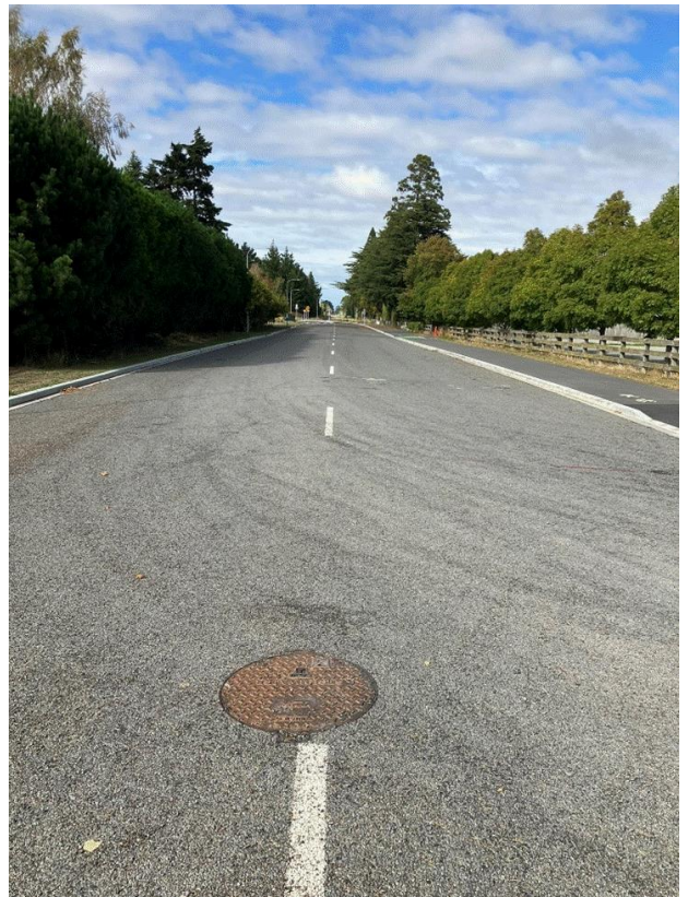
Plate 22: Stock water piped down the centre of West Melton Road
