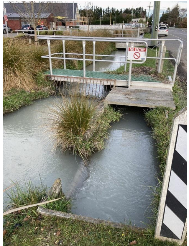
Plate 8: Existing debris grille on Weedons Ross Road
