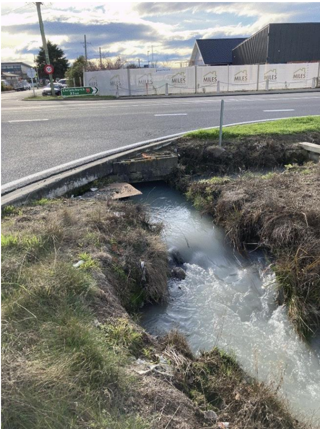
Plate 5: Existing outlet to box culvert under SH73
