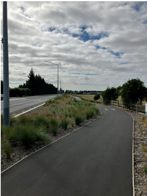
Plate 19: Shared user path and first-flush swales on SH73. Stock water piped along fence line.
