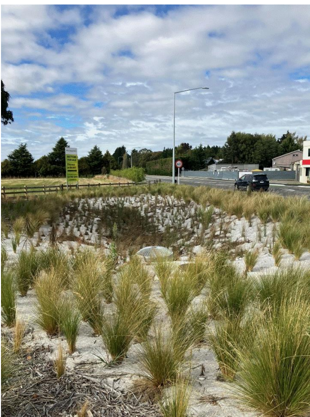
Plate 23: First-flush basin at SH73/Weedons Ross Intersection
