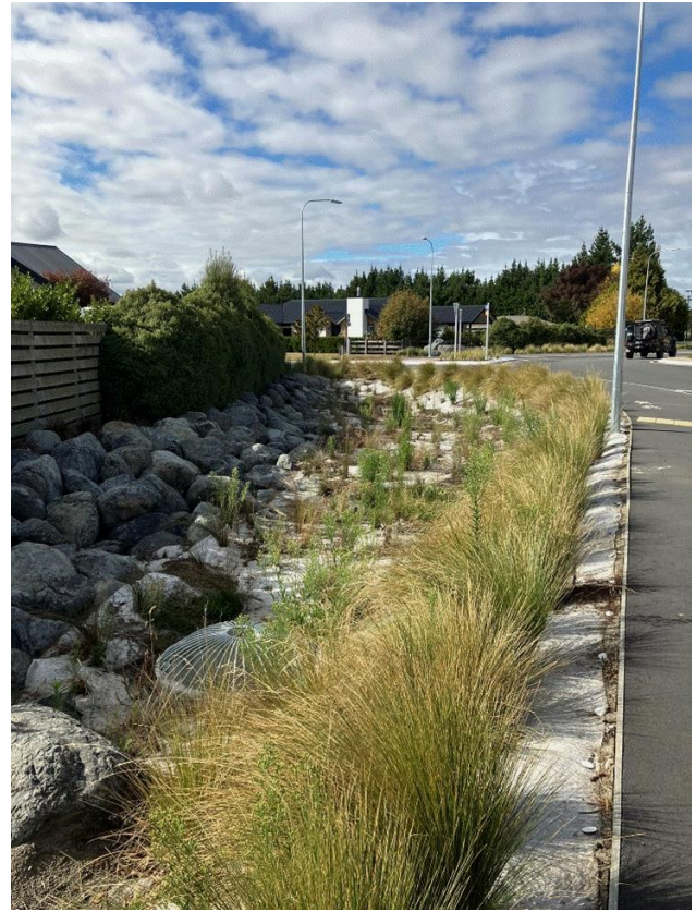
Plate 26: First-flush basin at the entrance to Kingsdowne Drive
