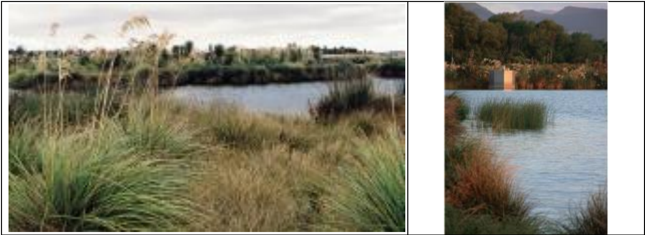
Figure 15 – Wigram East retention basin with a view towards the basin outlet structure (WWDG, 2009)
