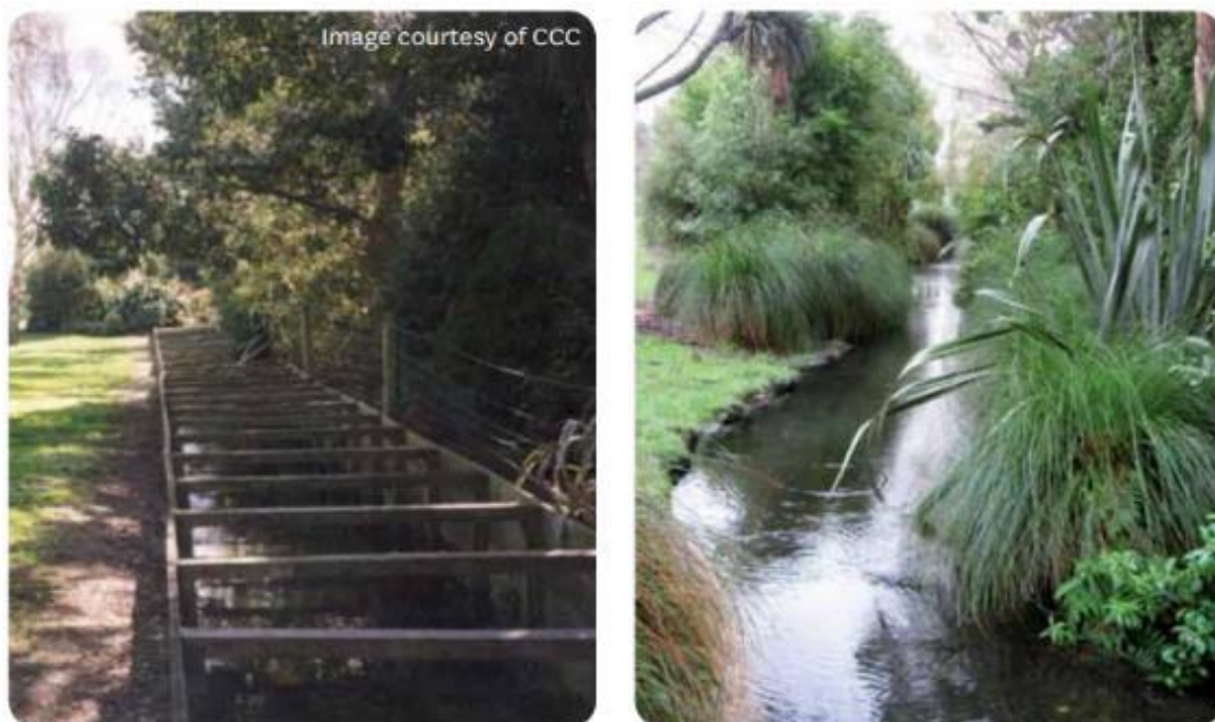
Figure 5 Papanui Stream in Erica Reserve – before (1999) and after naturalisation of the timber lined drains (in 2010) reproduced from updated WWDG (2010).
