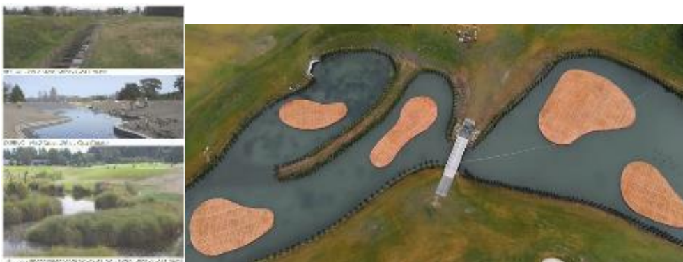
Figure 10 Stream naturalisation and inclusion of floating wetlands within the No.1 Drain, 2019 2 .
