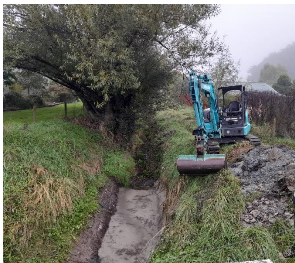
Figure 6: Excavation of sediment from Waipawa drainage channel
