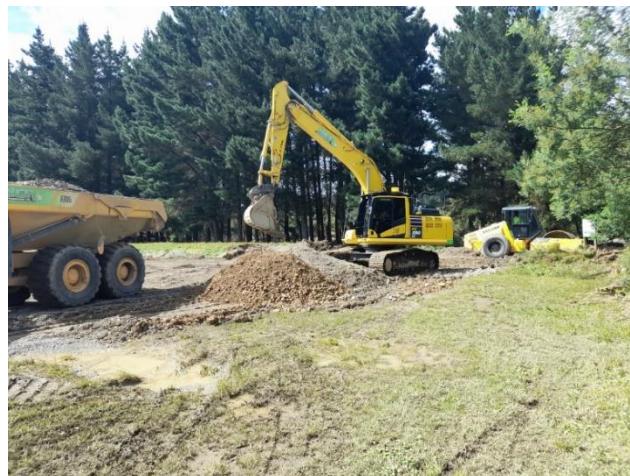
Figure 4 Waipawa stopbank rebuild
