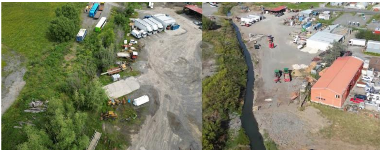
Figure 8 Clearing of willow-choked drainage channel
