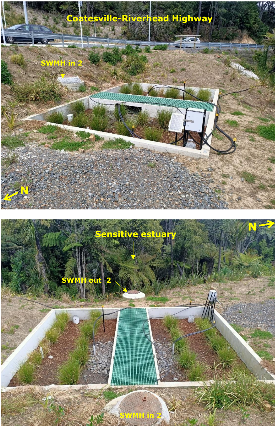
Figure 2 Annotated photographs to illustrate the site description and show the monitoring equipment of Figure 3. The stormwater manholes are labelled as SWMH in 2 and SWMH out 2 to provide context for Figure 4.
