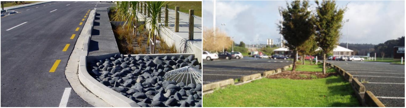
Figure 4: Example of a raingarden (left) and swale (right), (Auckland Council Raingarden Construction Guide and Auckland Council Swales & Filter Strip Construction Guide).
