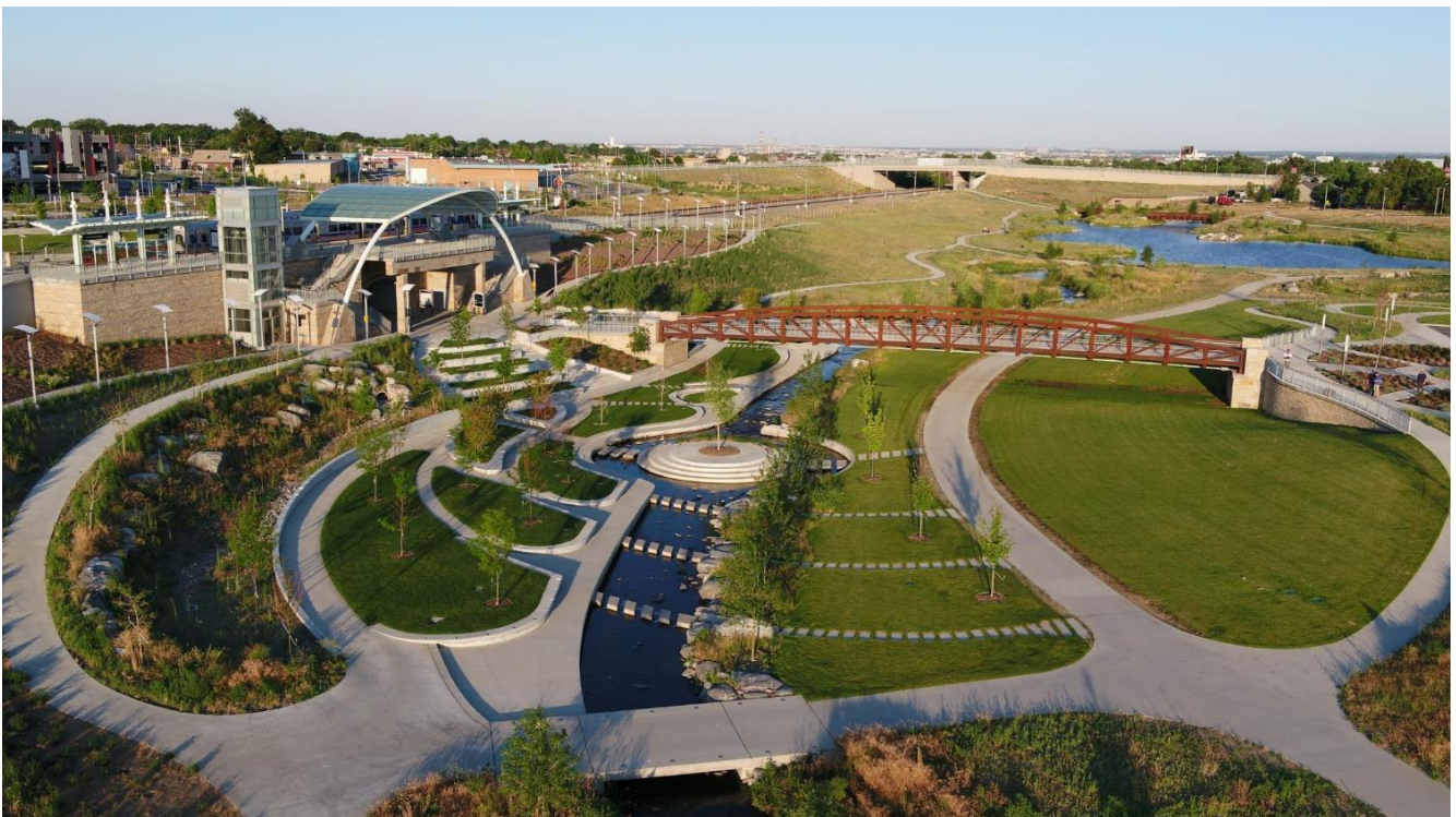
Figure 10: Westminster Station Park, Denver (Source: Mile High Flood District)
