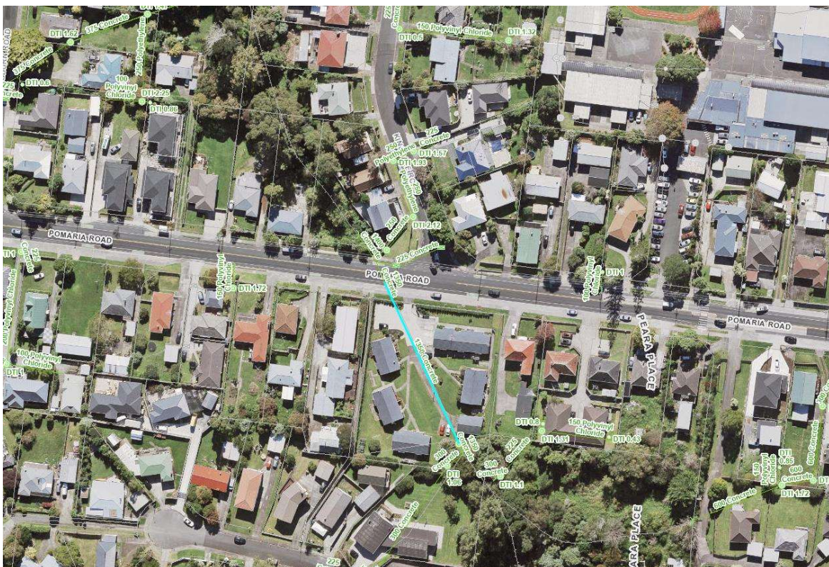
Figure 5: Pomaria Road Culvert
