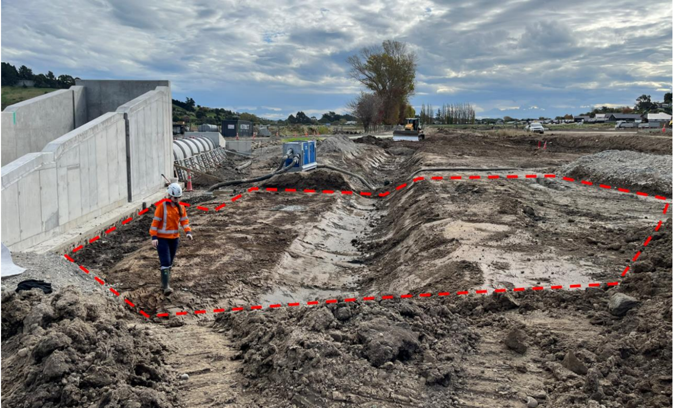
Figure 10. Exposed foundation at a scheduled inspection
