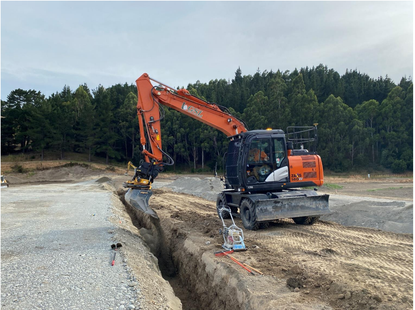
Figure 12. Trenching for chimney filter and placement of filter material.
