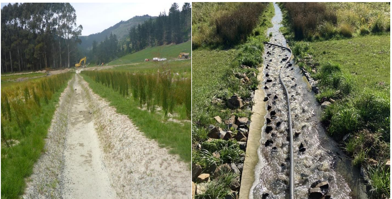
Figure 17 Two sections of the low flow channel. Left looking upstream towards forebay pond and transition. Right engineered grade transition between forebay pond and low flow channel during a small flood
