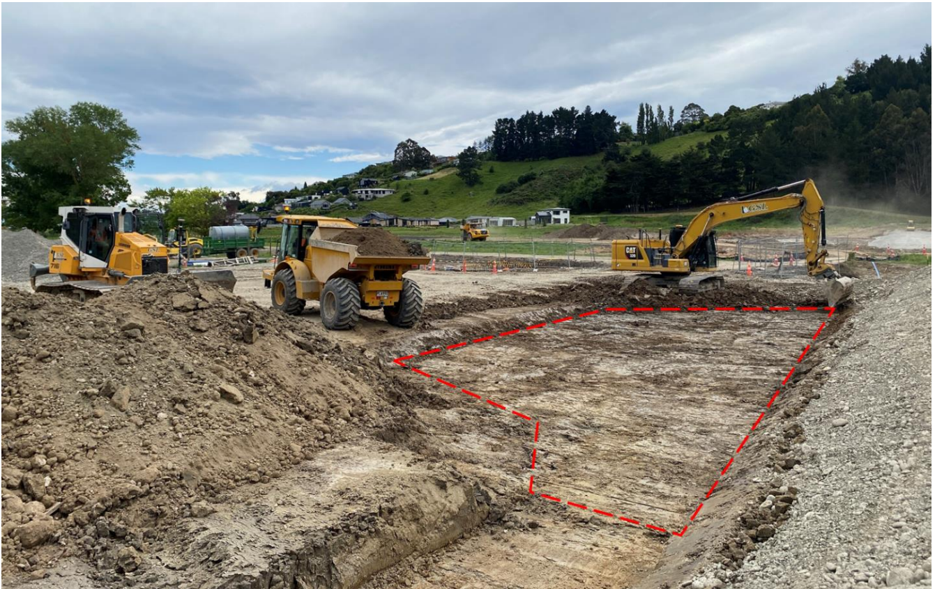
Figure 9. Exposed foundation prior to placement of core fill
