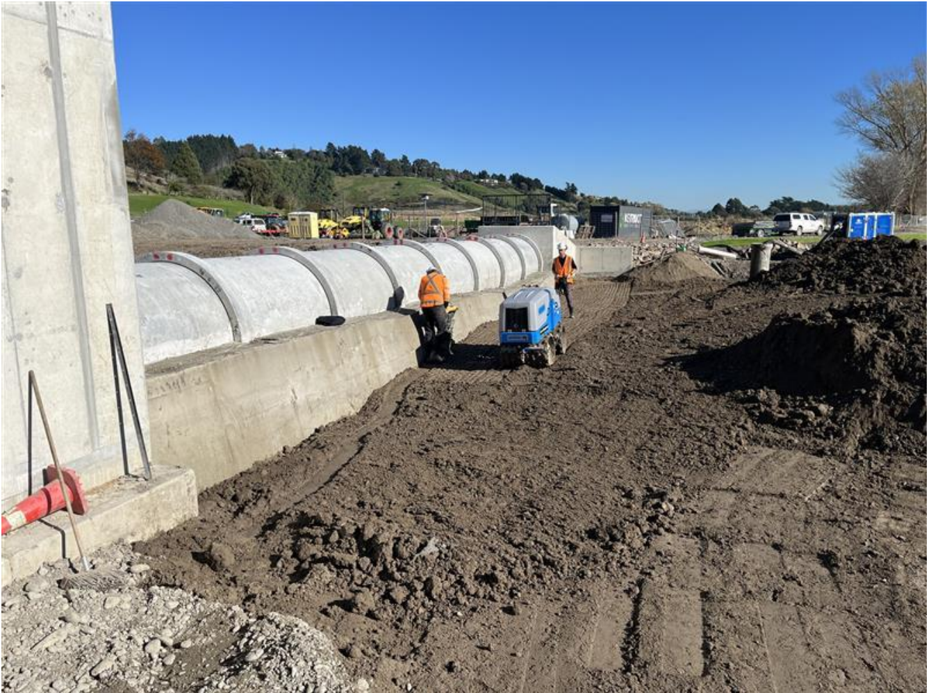
Figure 13. Compaction of core fill close to structures.
