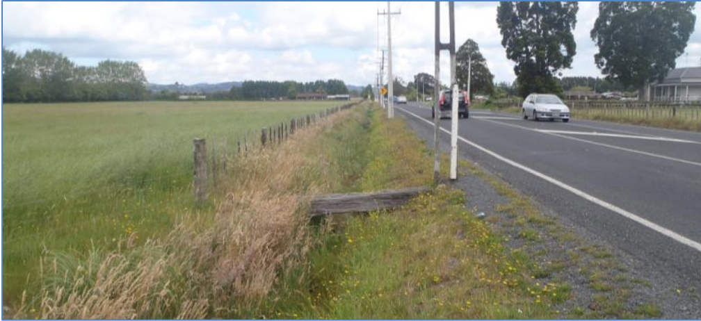
Figure 9: Cosgrave Road Table Drain
