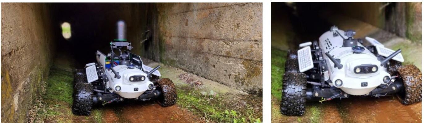
Figure 2: Pipe-i robotic scanner on a recent culvert monitoring project
