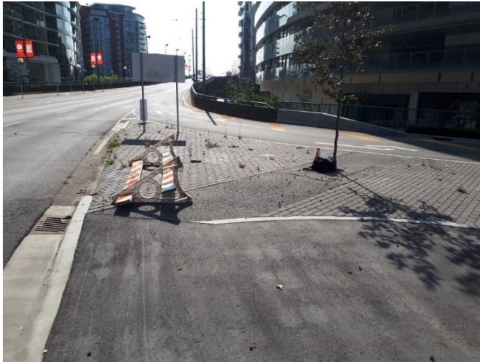
Photo of permeable pavement at Expo & Smithe, September 2020
