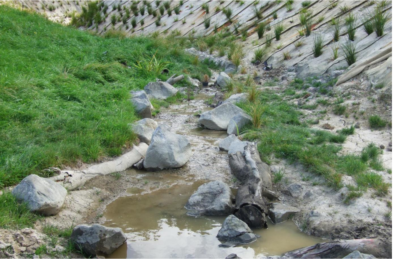
Photograph 5: Stream habitat (not completed) with trial diversion of flow through channel
