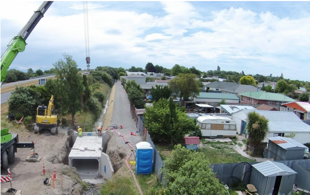
Photograph 1: Parnhams Drain upgrade works, Kaiapoi, December 2015
