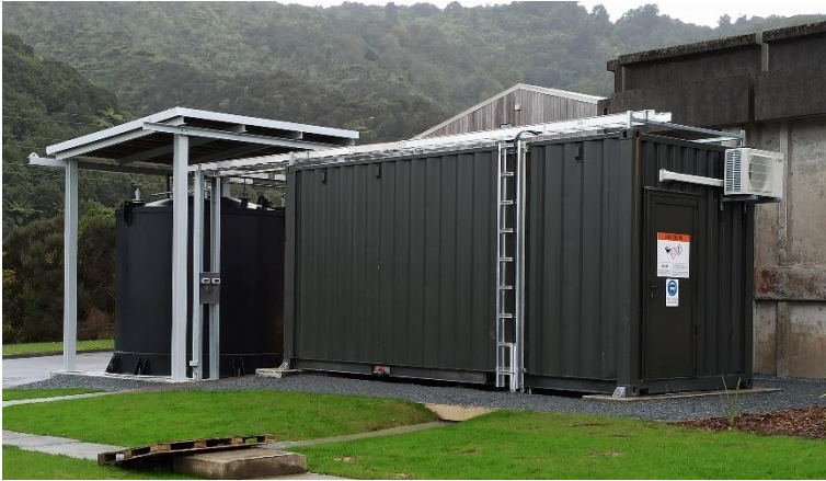
Figure 4: Te Marua WTP Fluoridation System
