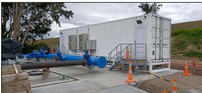
Figure 6: Containerised switchroom
