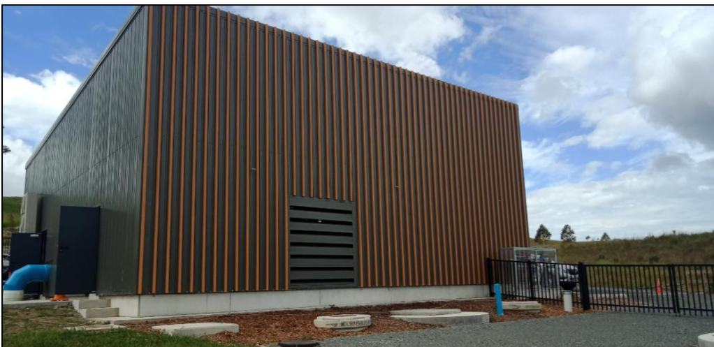
Figure 9: Completed lightweight structure (pump station building)
