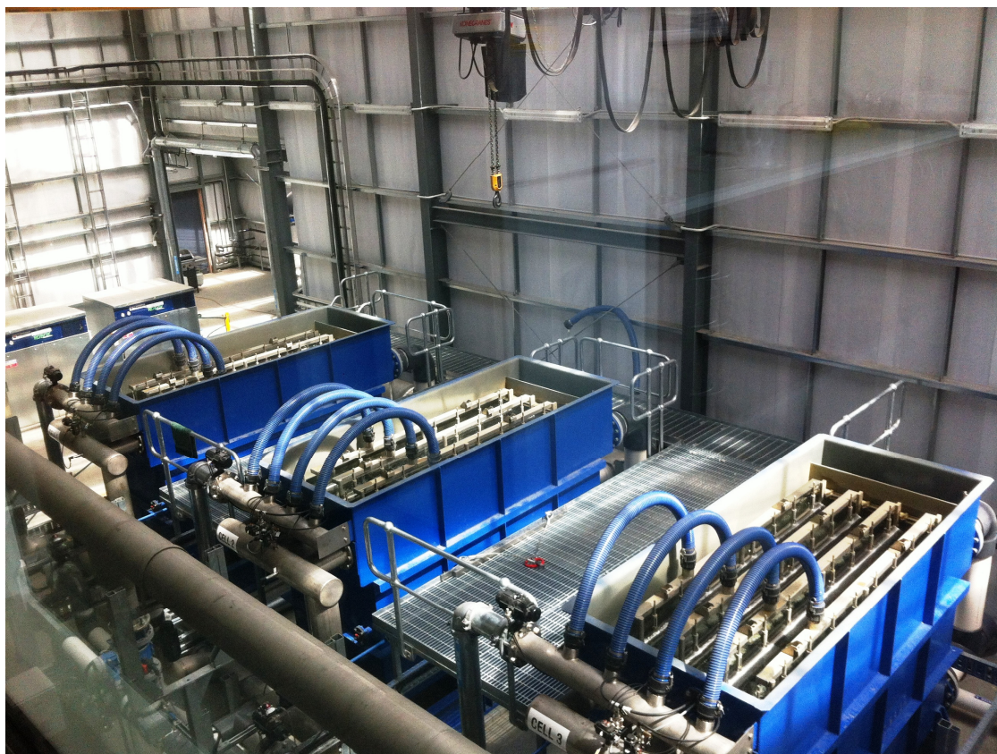
Photograph 6 – Construction of the Sludge/Backwash and CIP Tanks
