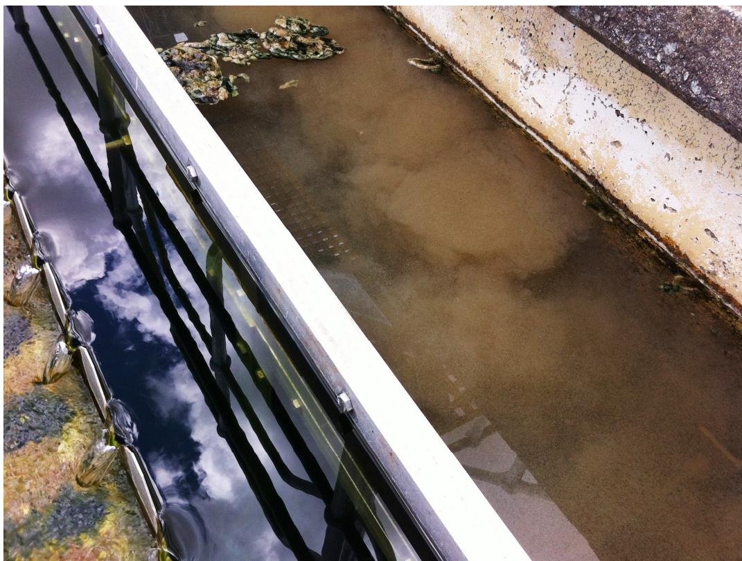
Photograph 9 – Clarifier Inlet February 2013
